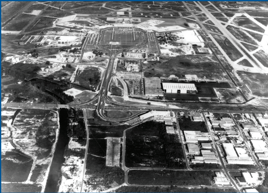
20th Street Terminal - 1959
