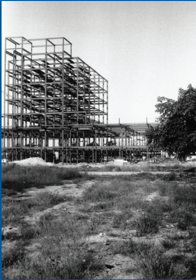
20th Street Terminal under construction - 1957
