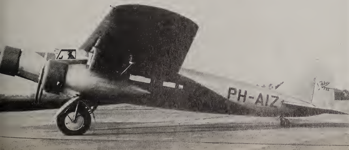
left The Fokker F.XX with Wright Cyclone engines, which appeared in 1933, was the most refined of the trimotor designs, with, for example, a retractable undercarriage. It carried twelve passengers
