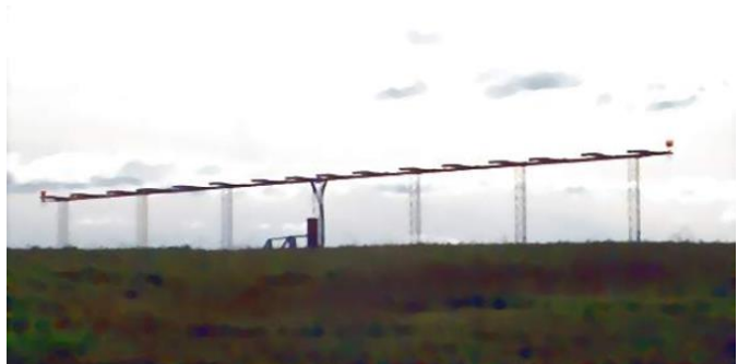
Figure 22. Localiser Antenna of an ILS
