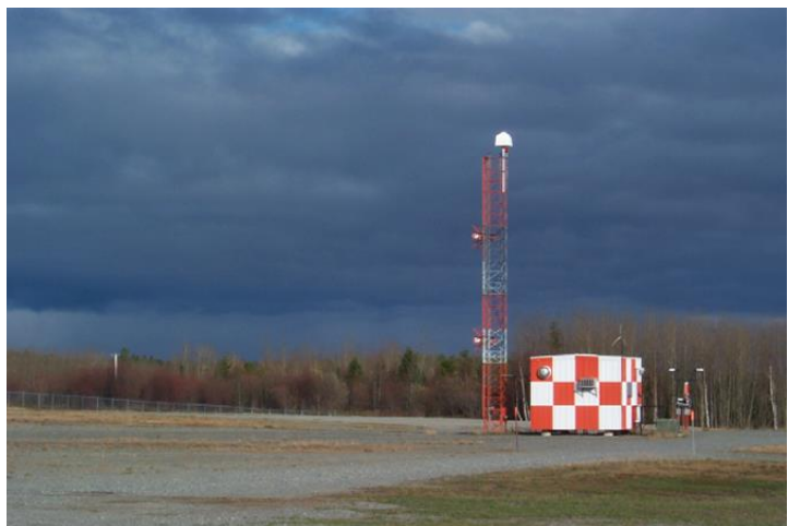
Figure 23. Glide Path Antenna of an ILS
