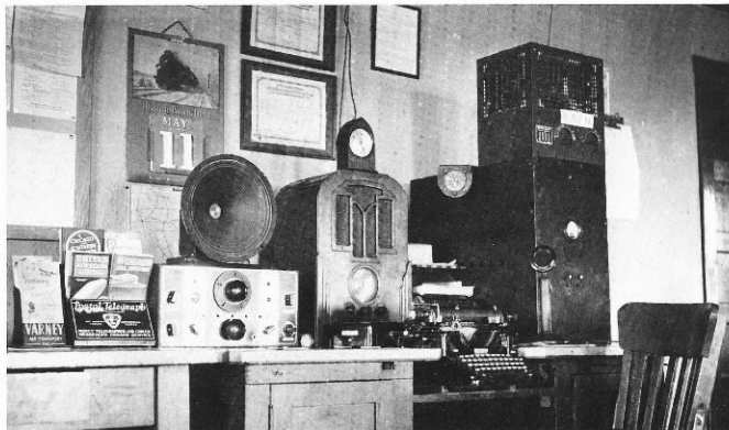
Communications in the early days left something to be desired, as shown by the station interior at Pueblo.
