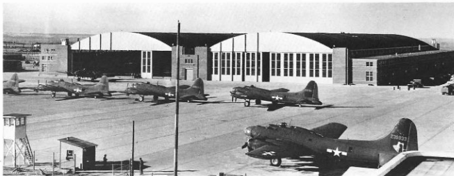
On October 1, 1943, the $5,000,000 Modification Center was opened at Denver. Some of the B-17 Flying Fortresses that were modified are parked in front.
